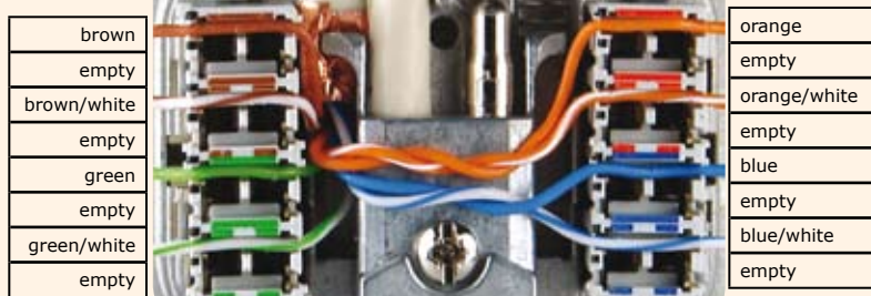
Fig.: Applying the wires
