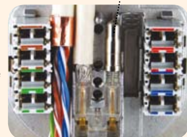
Fig.: Applying the cables
